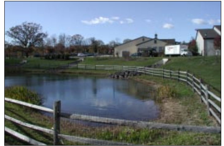
Wet detention basins planted with appropriate plant material can improve the look and function of the basin.
